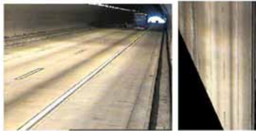
Figure 14: Example of a captured image (on the left) and the correspondent rectified image (on the right).
