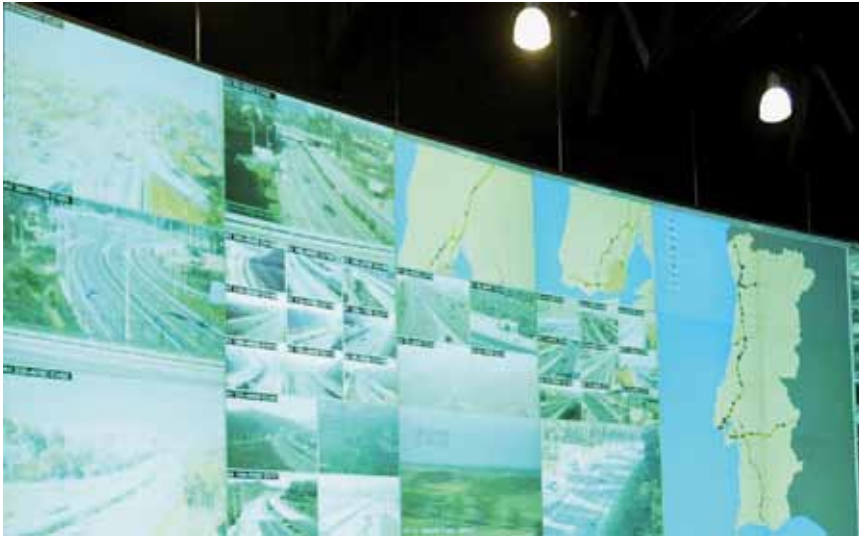
Brisa's Operational Control Center aims at guaranteeing new levels of road safety in the network, better traffic management and better traffic flow.
